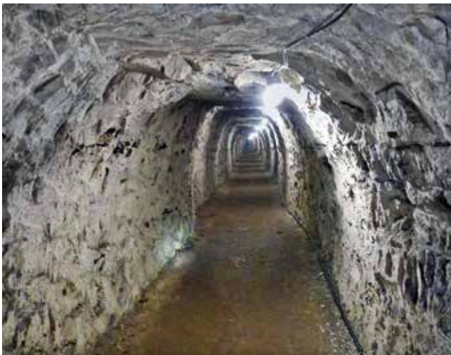
The chalk-cut ARP tunnel, close to its junction with the mainline tunnel. Photo Kenneth Barclay
